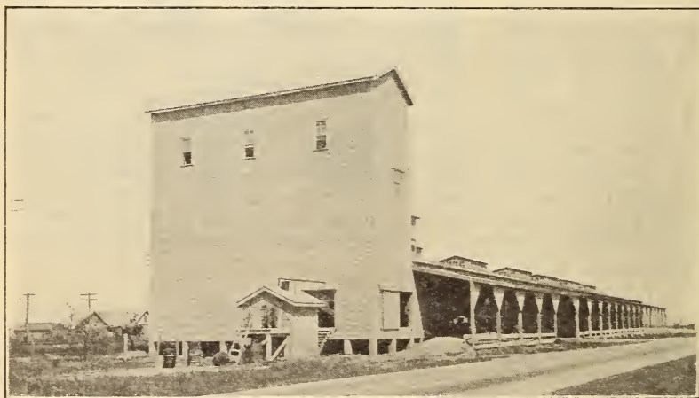
FIGURE 7.—Warehouse and drier installation, Nome, Tex.
